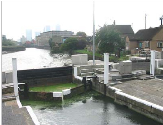
One of the locks has been blocked off with a steel barrier, but this can be lifted out to allow the lock to be used as intended.
