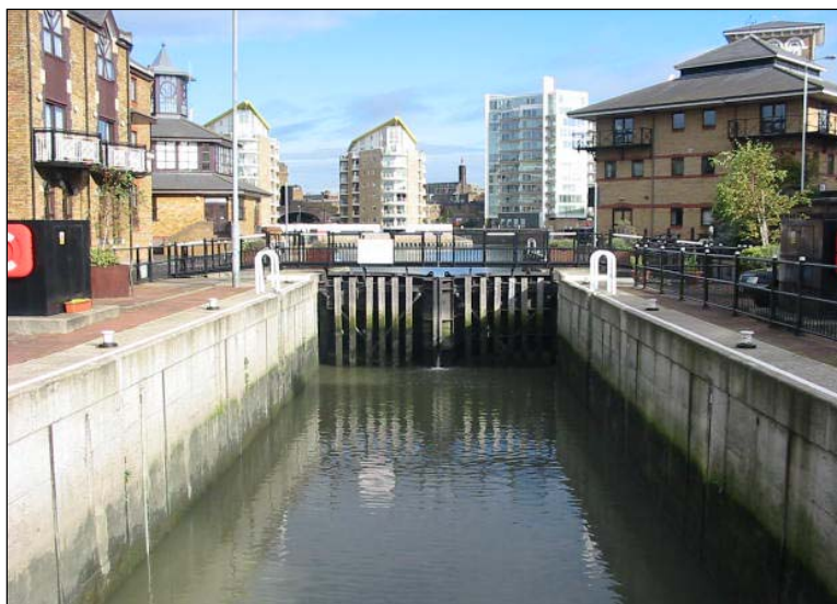
Entering the Limehouse Ship Lock from the Thames, and looking towards the basin. It can be seen how close the buildings crowd round the lock. It is still wider than many locks, but until a few years ago it was twice the size as very large ships entered the basin to unload to canal boats. The Regents Canal entrance is to the left across the basin, and the Limehouse Cut branches off to the right.
